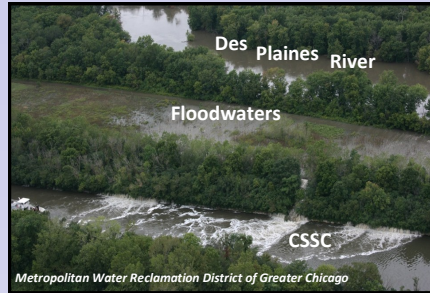
Des Plaines River floodwaters flow into the CSSC upstream of the electrical barriers (September 2008)
