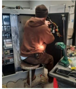
The newly redesigned control cabinet finally takes shape as Zach begins to connect wires to electrical components inside. Photos: Beth Glidewell/USFWS.
